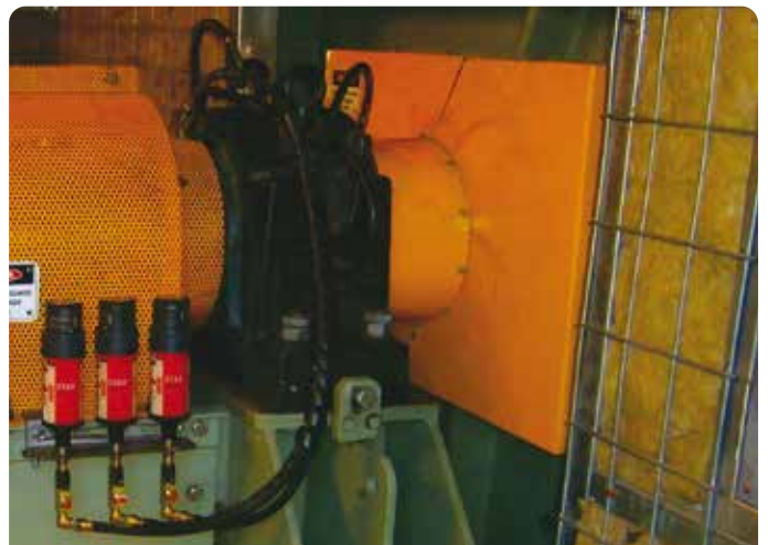
Application Fan support bearings Lubricator perma STAR VARIO L250 Installation kit K330
