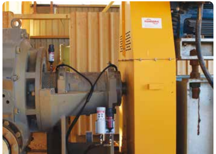
Application Horizontal slurry pump labyrinth seals & impeller mechanical seal Lubricator perma STAR VARIO L250 Installation kit K230C & direct mount
